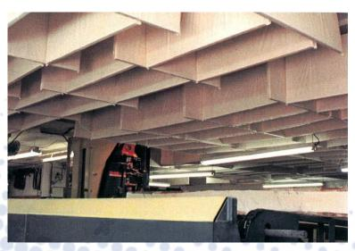
More than 600 Polywrapped Ceiling Baffles reduced overall noise levels by 8 dB(A) in this wood working facility.
